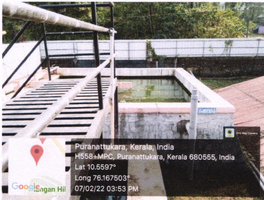
ACON, Clarifier, Water treatment plant
